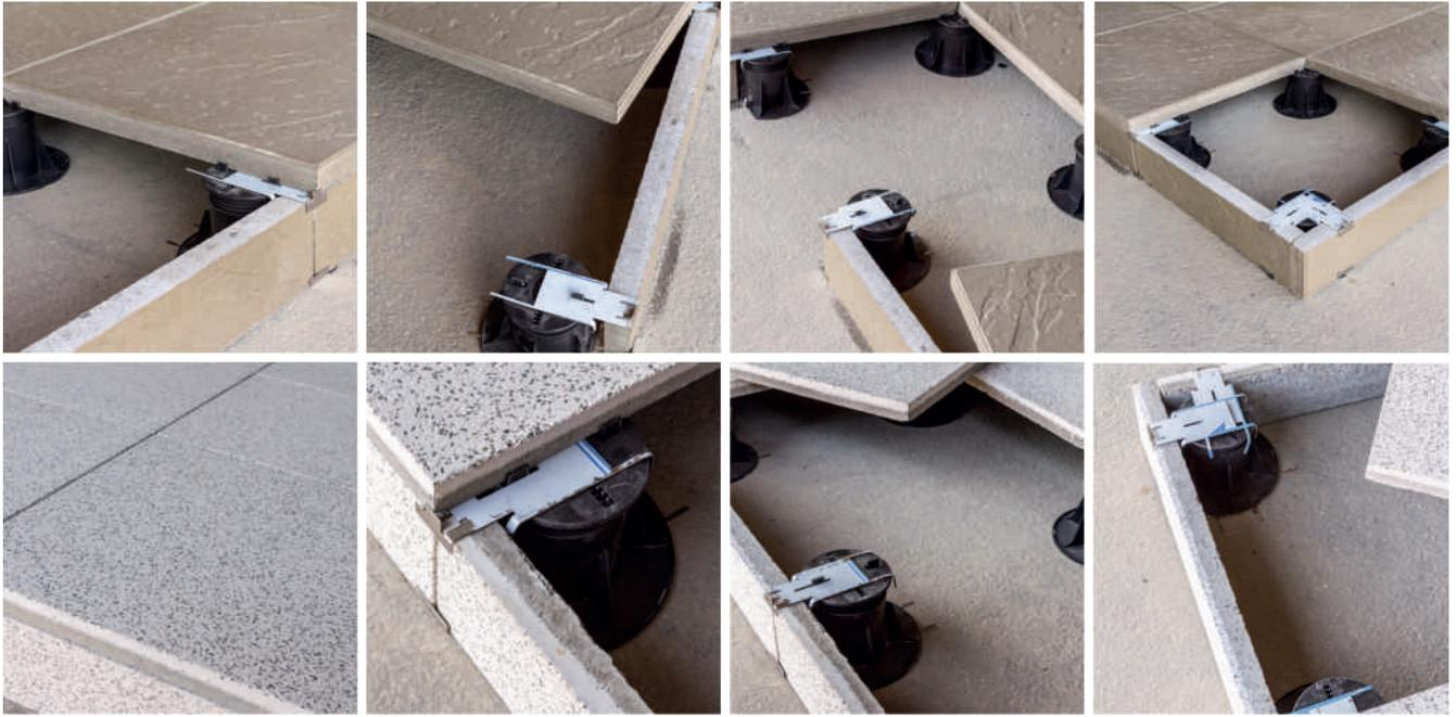
The use of clips is very simple both for the continuous face and for mounting the corner of the surface.
