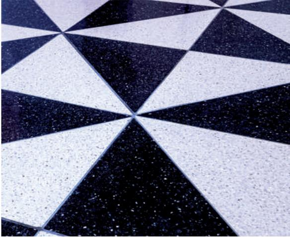
is a terrazzo paving in the shape of a right equilateral triangle according to the attached photo. It is a two-layer paving, where the upper visible layer is formed by terrazzo crumb of various drawings, colors and sizes, with the possibility of coloring into the mass. The lower, supporting layer is made of river gravel and Portland cement. Triangles are produced in two basic dimensions.
