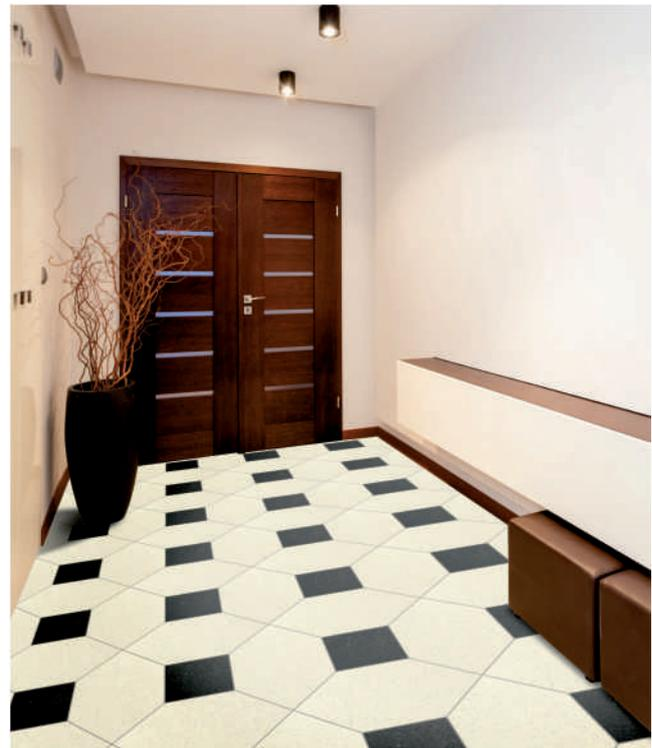
Another possibility of a non-traditional method of irregular hexagon laying is the use of the central beginning of installation (star design), and thus the creation of very interesting patterns in the laid floor area. The variability is again very high and the given limitations are given only by our imagination. One of the possible designs is in the attached photo and set.
