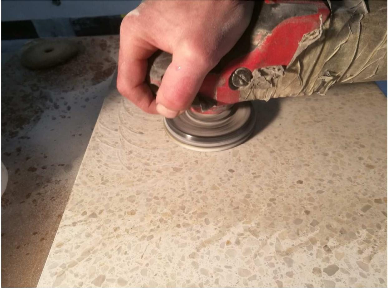
9. **Impregnation of the repaired Terrazzo element after repair** - let the repaired element dry - depending on the temperature approx. 30-60min. Subsequently, we impregnate the element, which closes the element against water and contamination. It is good to apply about 10 hours later or the next day one more coat.
