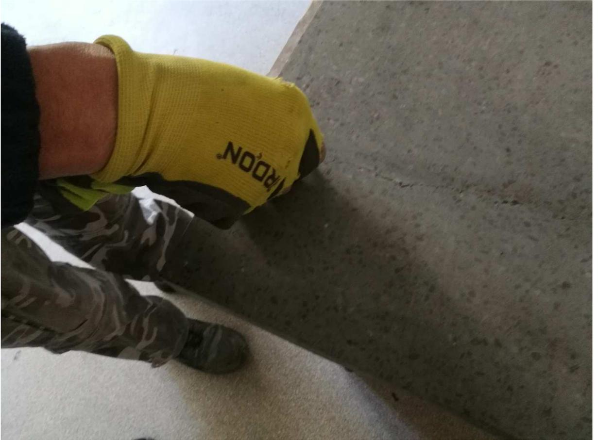
3. **Joint degreasing** - if the terrazzo element is already in construction, the terrazzo element's surface is greasy. The sealant would not properly anchor on this element. Therefore it is necessary to degrease the place of repair and jointing firstly. Degreasing is performed with ACETON thinner (acetone).
