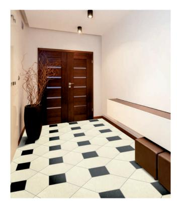
Another possibility of a non-traditional method of irregular hexagon laying is the use of the central beginning of instalation (star design), and thus the creation of very interesting patterns in the laid floor area. The variability is again very high and the given limitations are given only by our imagination. One of the possible designs is in the attached photo and set.
