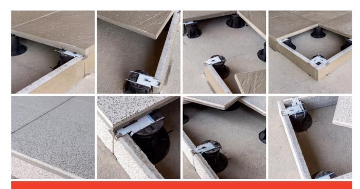
The use of clips is very simple both for the continuous face and for mounting the corner of the surface.
