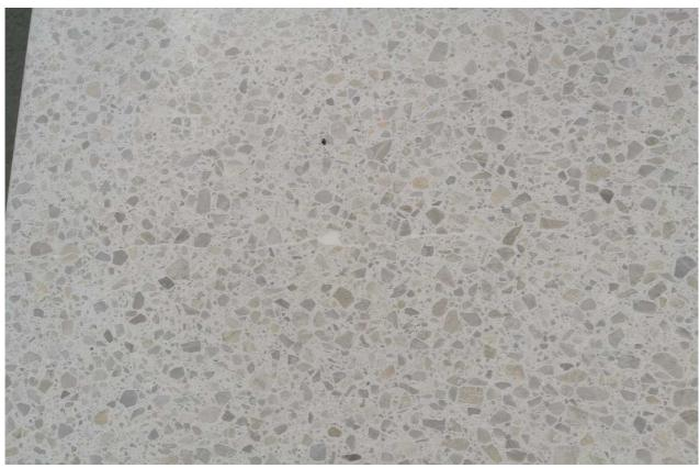
Photo repaired cracks - white terrazzo - the next day, photo close up - about 20cm
