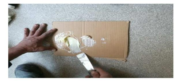
5. **Preparation of sealant** - always prepare such amount of sealant that after mixing with hardener we are able to process in approx. 10 minutes = push into cleaned cracks. The hardener / putty ratio is according to the instructions. Subsequently, the sealant hardens and its processing - pressing into the joint, becomes impossible. Care must be taken to properly mix the putty and hardener into the entire amount of putty.
