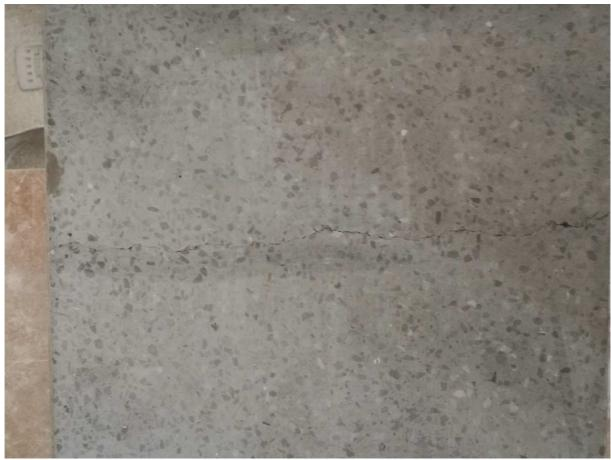
2. **Preparation for repair** - cleaning the joint - the crack on the construction site is usually already filled with dirt, which is clogged into a thin capillary crack clogged with water when cleaning. Therefore, it is necessary to mechanically remove this dirt from the joint. Removal is carried out for example with a thin breaking knife in the direction of the joint.
