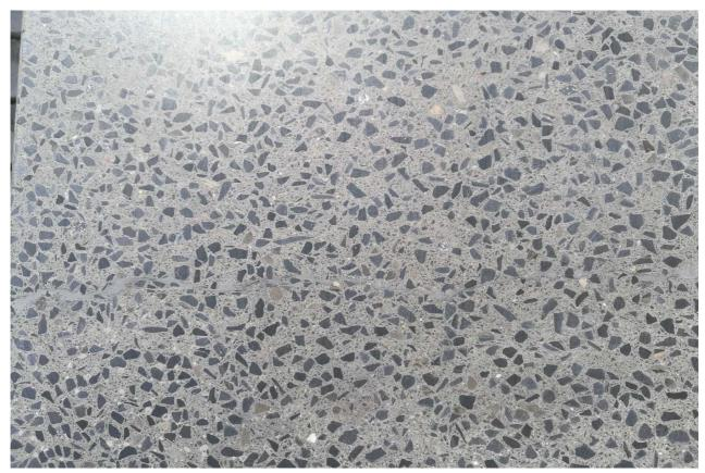
Photo repaired cracks - black terrazzo - the next day, close up - about 20cm
