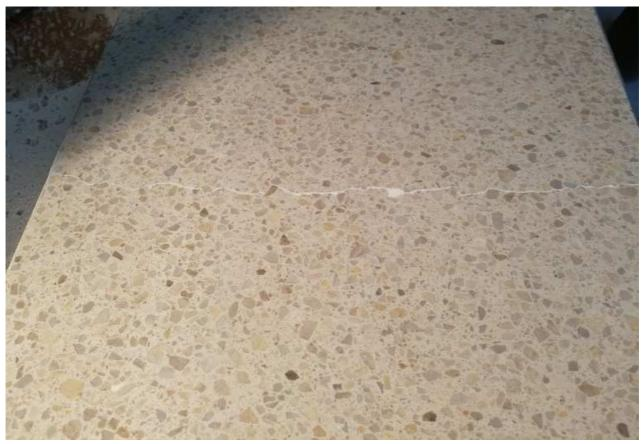
Photo of repaired joints in the terrace immediately after repair - wet surface
