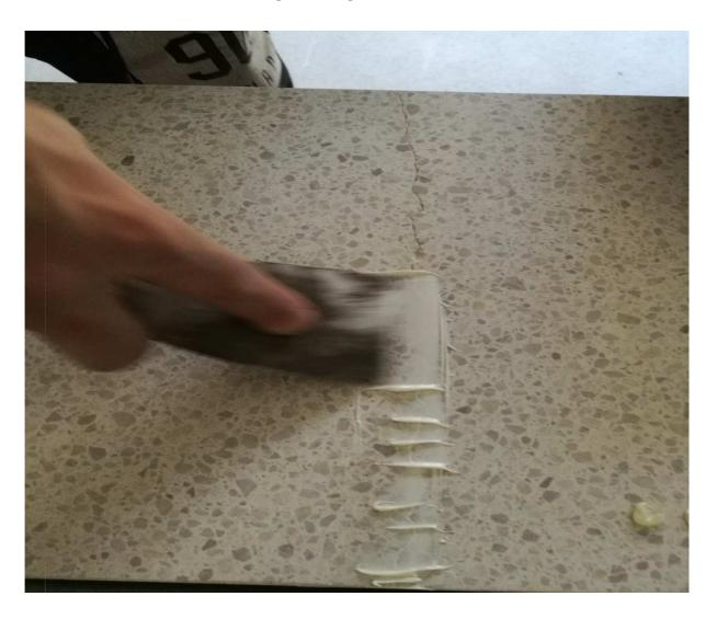
7. **Grinding of putty** - normally putty on the surface of the element is hard for grinding after about 30-45 minutes. Grinding is usually carried out by dry sandpaper so that all the sealant on the element top is removed. The terrazzo element is then cleaned of dust. The advantage is to work with the grinder with dust extraction - we did not have it for the test.
