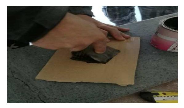
6. **Applying the sealant into the joint** - the sealant is pushed into the joint in the transverse direction - perpendicular to the joint, several times in the same place, so that the joint is well filled. We try to keep the sealant layer as thin as possible on the surface of the element - we have to grind this layer of sealant, which is unnecessary costs.
