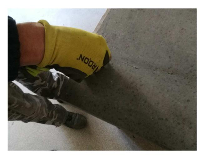
3. **Joint degreasing** - if the terrazzo element is already in construction, the terrazzo element's surface is greasy. The sealant would not properly anchor on this element. Therefore it is necessary to degrease the place of repair and jointing firstly. Degreasing is performed with ACETON thinner (acetone).
