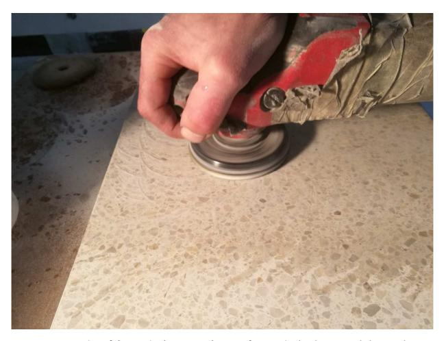
9. **Impregnation of the repaired Terrazzo element after repair** - let the repaired element dry - depending on the temperature approx. 30-60min. Subsequently, we impregnate the element, which closes the element against water and contamination. It is good to aply about 10 hours later or the next day one more coat.
