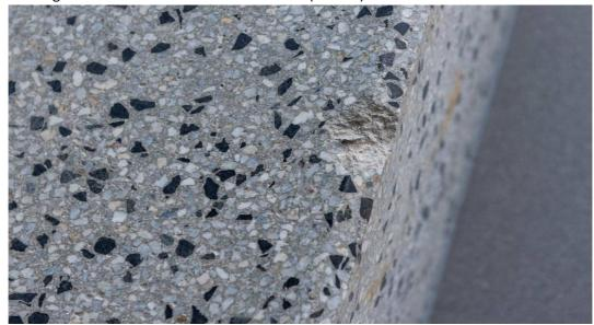
2. Reparation - the broken area must be carefully mechanically cleaned and loose particles removed. If the place is dirty, it is necessary to wash it with a wire brush. If it is greasy - for some reason, the damaged area must be degreased. This procedure is very important for connecting the repaired concrete mix
