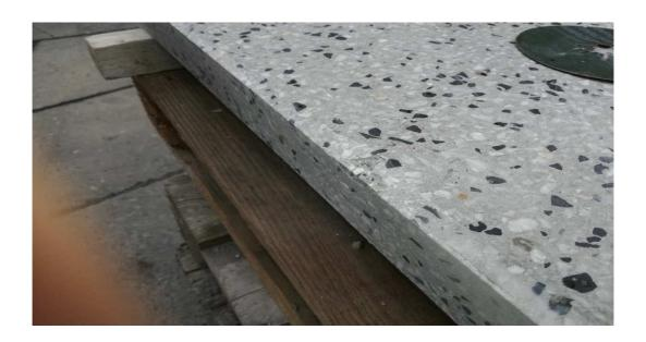
8. We finish the repaired place by fine grinding to the quality and fineness of grinding of the whole terrazzo element. We use the same fineness of sandpaper. The fineness of 100 - 200 is most often used for terrazzo products.
