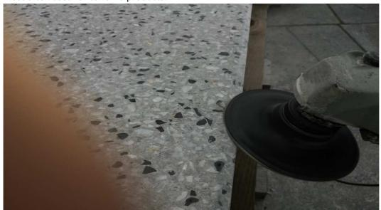
9. The repaired area is then impregnated together with the entire terrazzo element – see the picture
