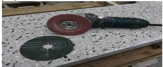
7. By grinding with a diamond wheel, we grind the repaired place to the level of the surrounding element, see photo 17 and photo 7. If there is an air bubble or pore at the repaired place, we recommend tamping the said bubble or pore with cement paste before fine grinding
