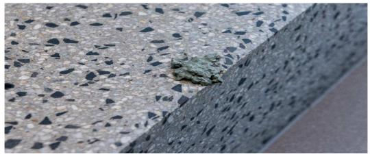
4. After applying the terrazzo mix, it is necessary to cover the repaired area with a piece of PVC foil so that the concrete mix used for the repair does not dry out quickly. The PVC foil is
