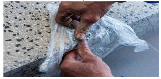
5. After two to three days, the foil can be removed and rough grinding can be started. The mixture used for the repair should be hardened and compact
